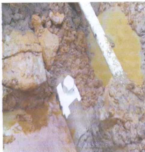
Fig C: picture taken after wrapped.
