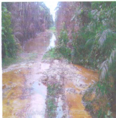
Fig D: picture taken after backfilled.
